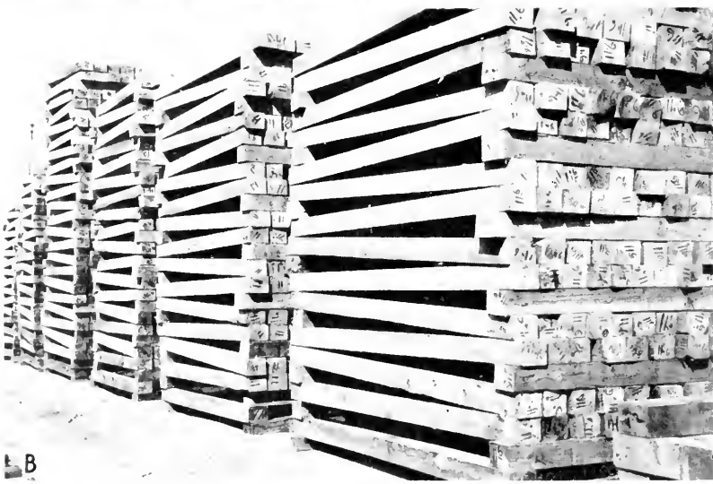
Railway cross-ties piled for air seasoning: A, Solid piling with 11 by 11 layers; B, a common form of open piling; the illustration shows 10 by 1 layers
